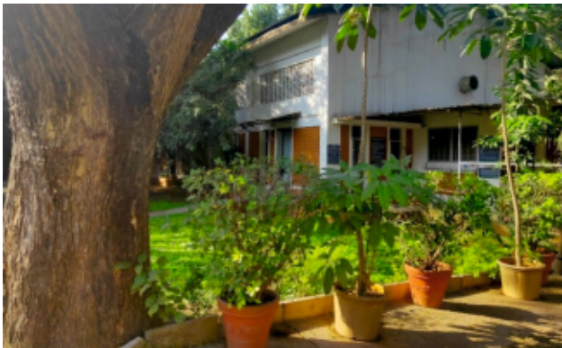
Dhamma Punna Vipassana centre at Swargate, Pune. Several such Vipassana centres were established by skillfully using different positions in Govt
